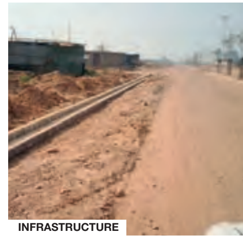
INFRASTRUCTURE 24 mtrs. wide road
