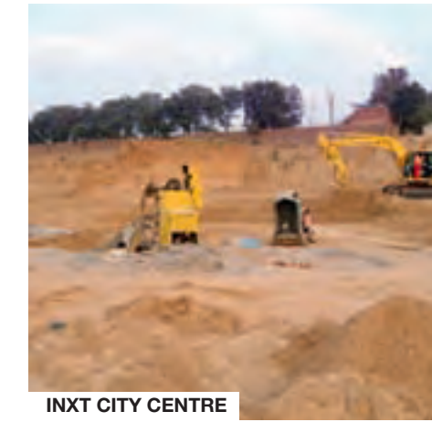
INXT CITY CENTRE Excavation
