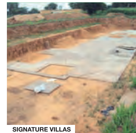
PCC in progress
