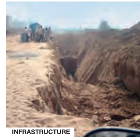
INFRASTRUCTURE Service work
