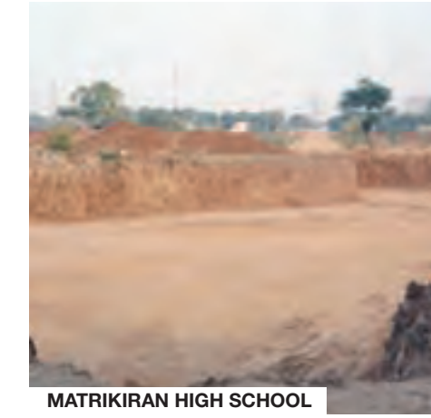
MATRIKIRAN HIGH SCHOOL Excavation
