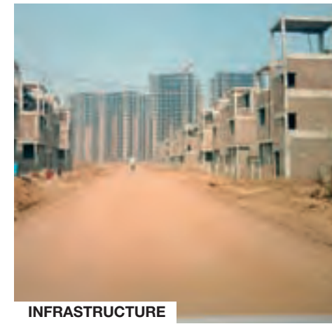
INFRASTRUCTURE 12 mtrs. wide road
